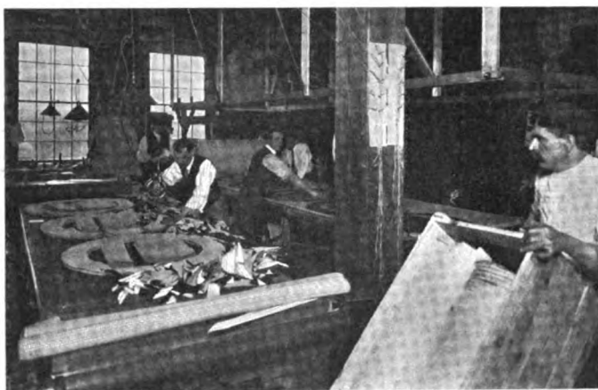
Hopewell Cutting Room, Cutting Machine In Action
